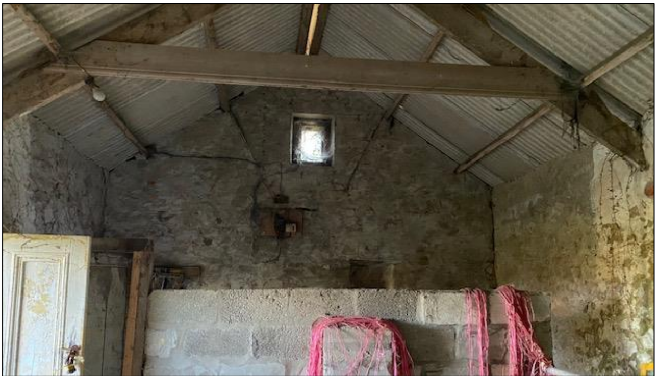
Figure 3. Internal view of the southern gable end of the barn.
