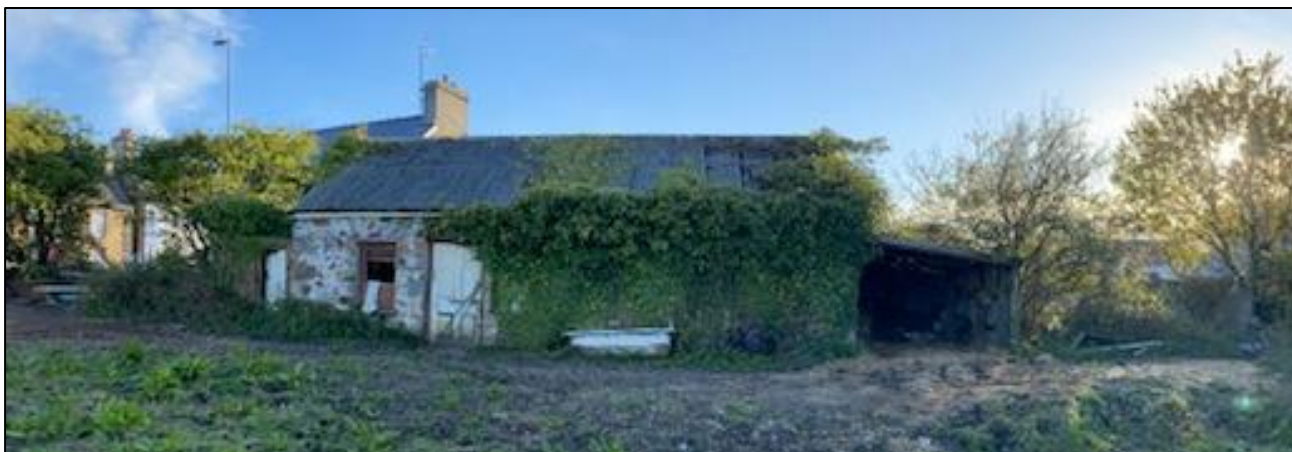
Figure 1. Eastern aspect of the barn.
