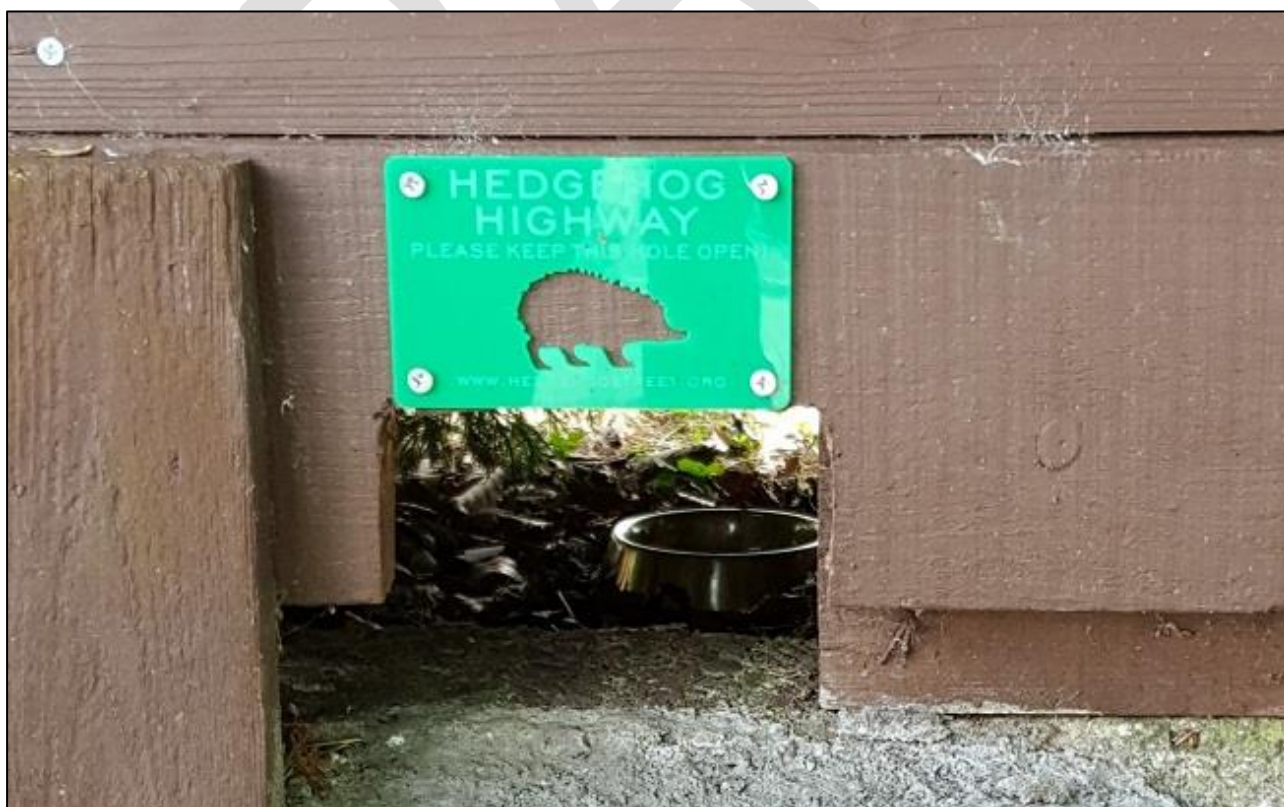
Figure 14. Hedgehog highway included in base of fence to allow hedgehog movement.
