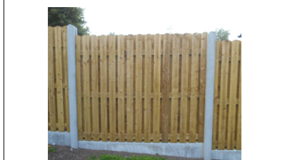
Product :- Hit & Miss Fencing Company:- TBC Colour:- Natural with Concrete Post
