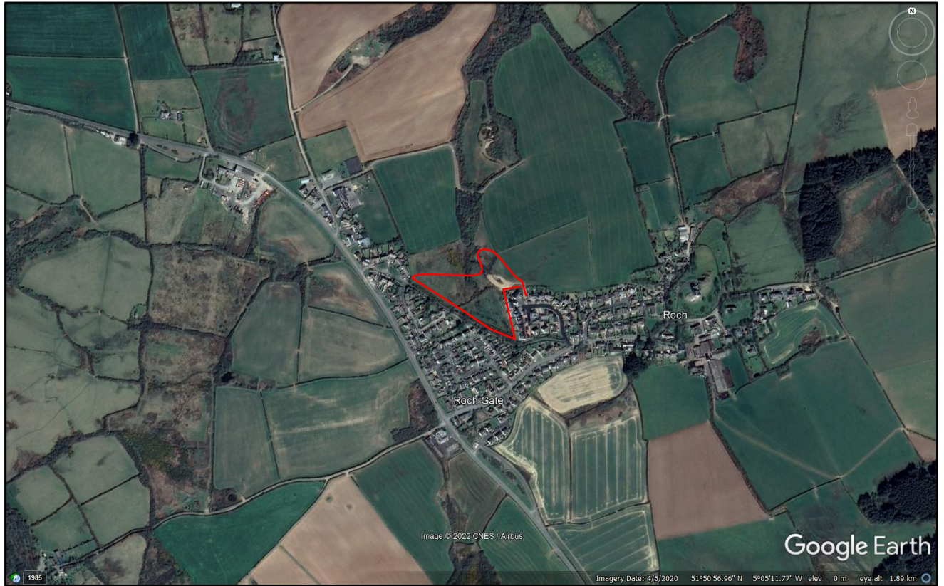
Figure 7. Aerial photograph of the site in relation to surrounding land use.
